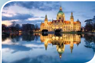
Headquarters Hanover, Germany
